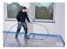
Subsequently, lay the pipe tension-free from above in a large arc according to the manufacturer's instructions.
