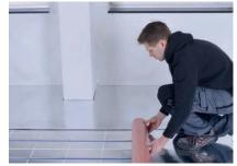
Lay the CompactFloor DIRECT 1.5 length for length tension-free. Joint edges should not overlap in the process.
