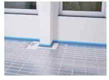
Lay a suitable pressure-resistant dry-construction floor heating and adhere the entire surface to the subsurface.
