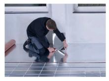
Cut out the individual cutouts in the room using a cutter or carpet knife.
