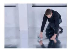
Adhere all joint edges using CompactFloor DIRECT 1.5 aluminium adhesive tape for sealing and optimum heat transfer.
