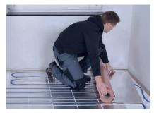
To lay the CompactFloor DIRECT 1.5 in a room, begin in a corner with the aluminium facing upwards.
