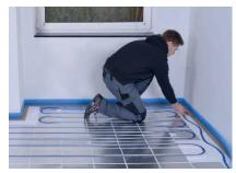
Cut off the edge insulating strips flush with the floor heating prior to laying the CompactFloor DIRECT 1.5.
